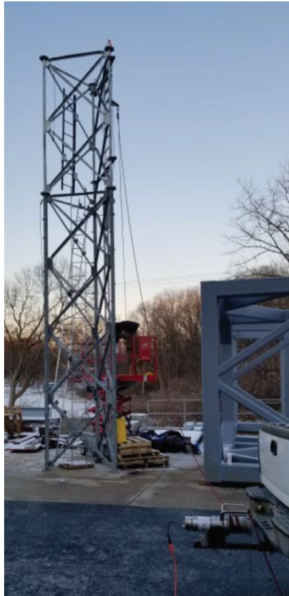
Tower and Capstan Set Up
